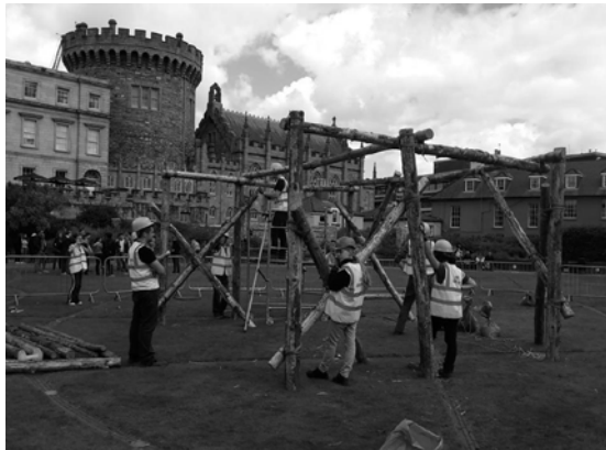
Figure 6. Working to build Casino Marino Project, Dublin Castle, 2014.
