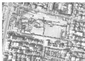
Figure 2. Treska factory site: existing situation 2014
