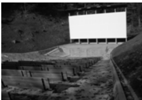
Figure 10. Arch. Kazimir Ostrogović: 1952 Summer theatre, Dubravka`s Promenade, Tuškanac, Zagreb (renovated in 2008)
