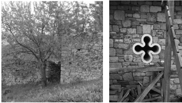
Fig. 7: Material displacement/replacement: stones from the old village houses in the church wall.
