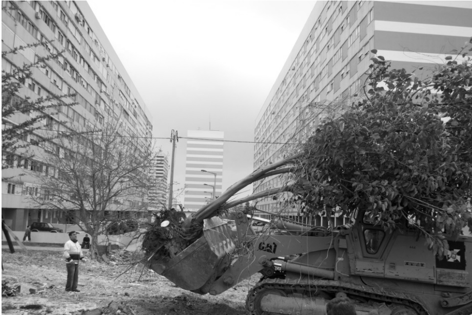
Figure 5. Transplanting trees, during demolition
